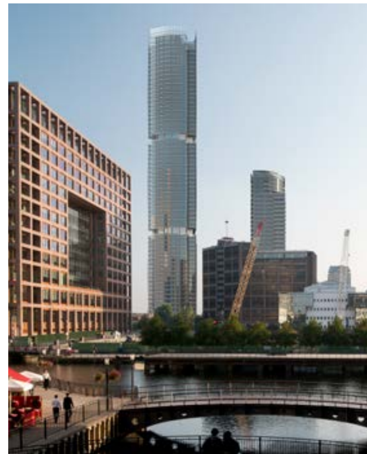
— Alpha Square, Canary Wharf Soaring up and out of the skyline, Alpha Square is a future landmark property for Canary Wharf.
